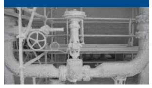
This control valve photo was taken in January when the temperature was minus 21 Celsius. It illustrates why remote, online monitoring and diagnostics is important to operators at a petrochemical plant in Canada. With a 667 actuator and a FIELDVUE DVC6200-AD instrument, the Fisher ET recycle valve assembly provides reliable flow control for water lines near the cooling towers.
