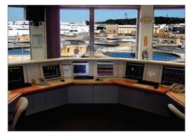
The integrated control system architecture for water/wastewater industries often incorporates a SCADA system for wide-area monitoring and control of operations from a single location. These operations may include remote pumping stations, wastewater collection systems, water distribution, sewer diversion, wet weather overflow protection, and weather monitoring. *Photo by Emerson Process Management*
