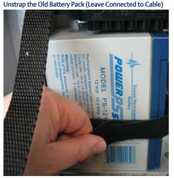
6. Place the old battery on top of the flow computer enclosure and place the new battery next to it.
