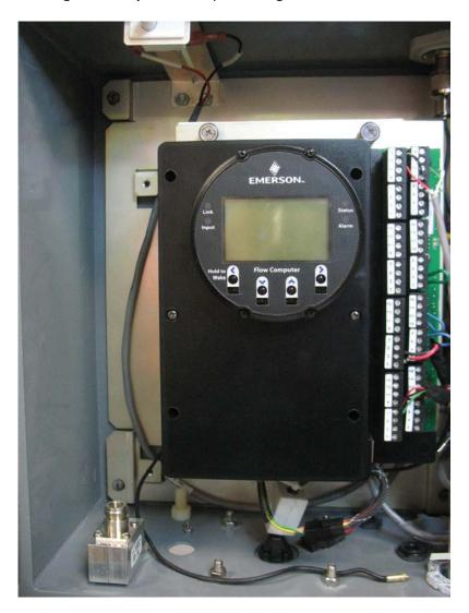
2. Remove power by unplugging terminal block TB2 (pins 1,3,5,7).
