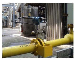
Wireless gas flow measurement with Rosemount Conditioning Orifice Flow Meter and THUM was easily integrated into the plant DCS.
