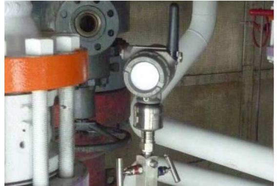
*The Rosemount 3051S Wireless Pressure Transmitter used to wirelessly measure flowing pipeline pressure.*
