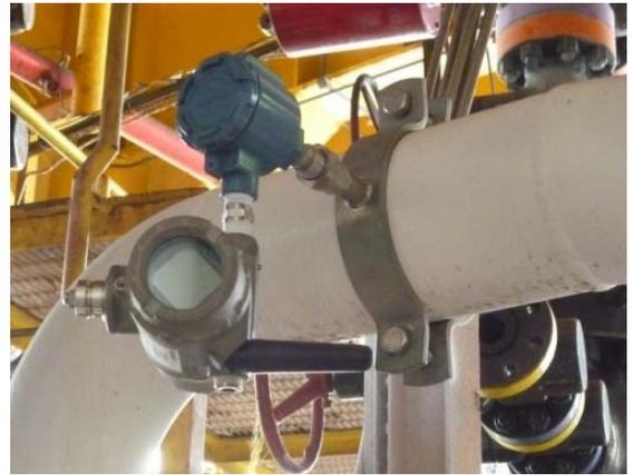
*The non-intrusive Rosemount Pipe Clamp RTD Sensor measures pipe surface temperature in the flowing lines.*
