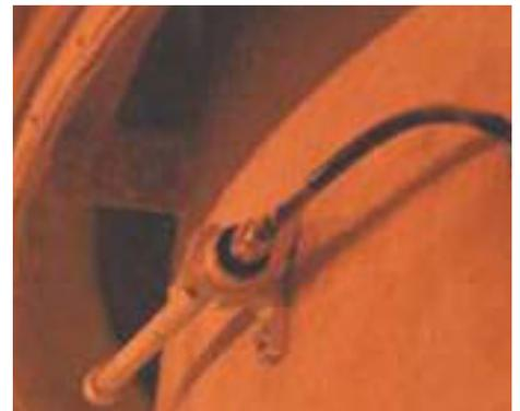
**Image 6.** A remote antenna on the center rotating shaft inside the sugar silo allows the wireless instruments to communicate with the Wireless Gateway located outside each silo.
