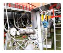
Emerson Smart Wireless Gateways were simply added to the existing Modbus network to make data from the wireless transmitters available within the existing control system.
